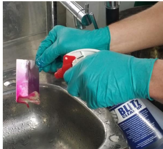
Neutraliser being sprayed onto cleaned weld
